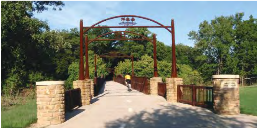
Pedestrian bridge as gateway feature
