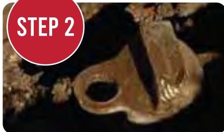
There is a single valve in the meter box. There is an arrow on top of the valve. To turn the water off, turn the valve one half turn clockwise until the arrow faces away from the meter. To turn it back on, turn it one half turn back towards the meter.
