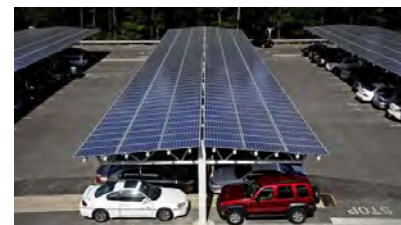
Solar panels incorporated into parking shade structures
