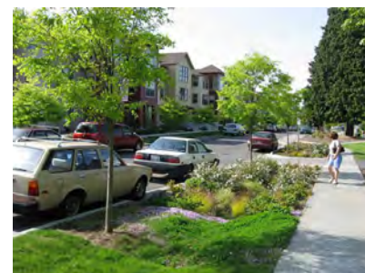
Stormwater feature - grassy swales
