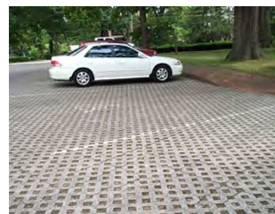
Stormwater feature - permeable pavement
