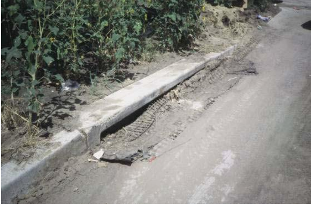
CLOGGED INLET PROTECTION IN NEED OF MAINTENANCE
