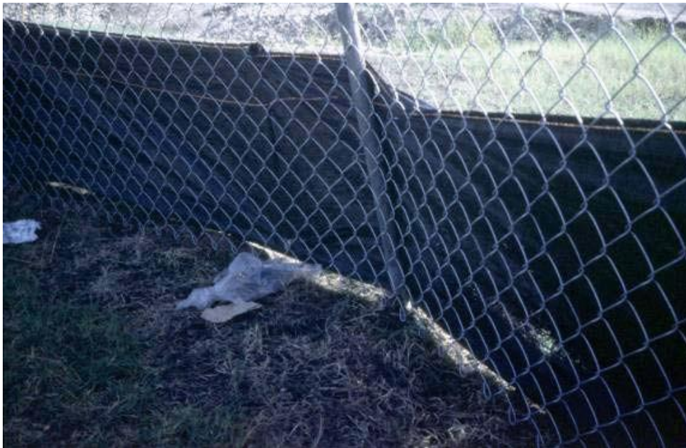
IMPROPERLY INSTALLED SILT FENCE. NOTE GAP BETWEEN FENCE AND GROUND
