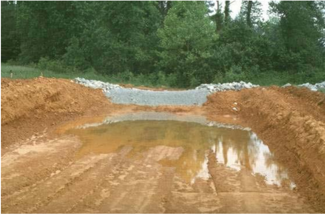
STONE OUTLET SEDIMENT TRAP
