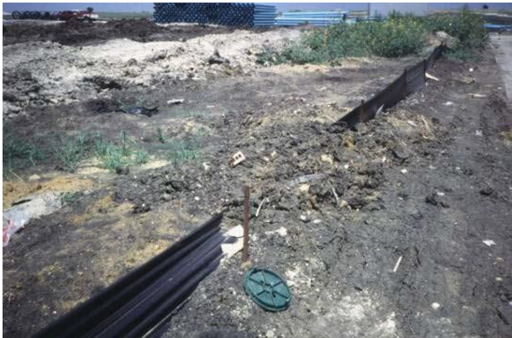
DAMAGE DUE TO CONSTRUCTION TRAFFIC & DUMPING
