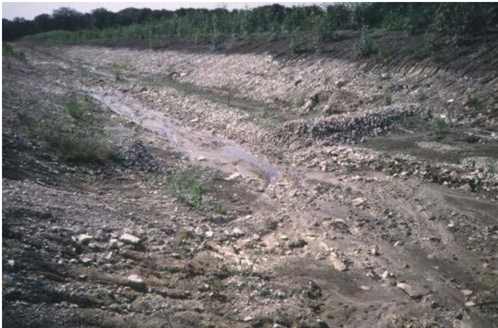
FAILED CHECK DAM DUE TO IMPROPERLY SIZED RIP-RAP
