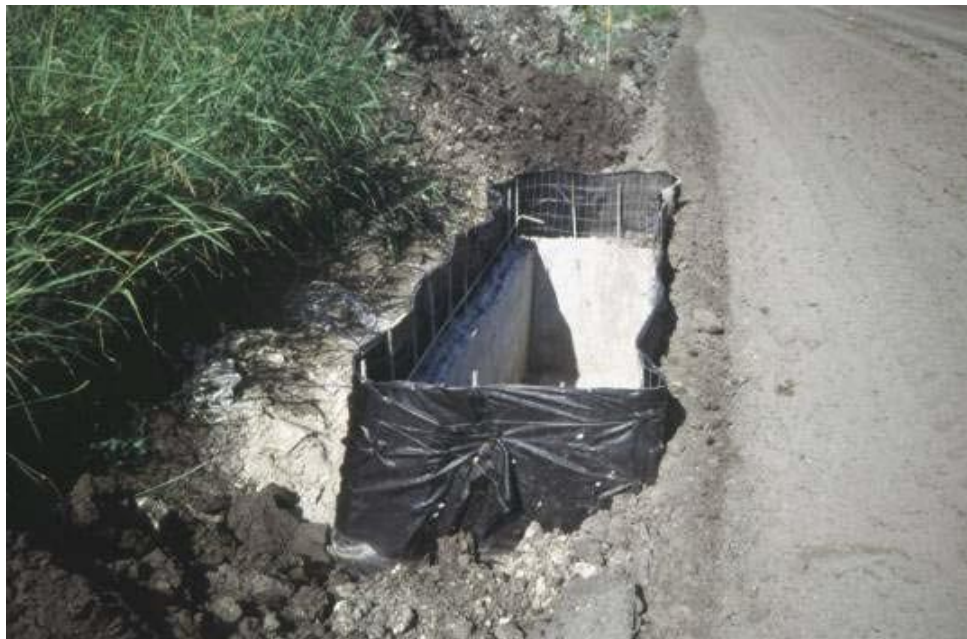
PROPERLY INSTALLED FILTER FABRIC ON UNFINISHED CURB INLET
