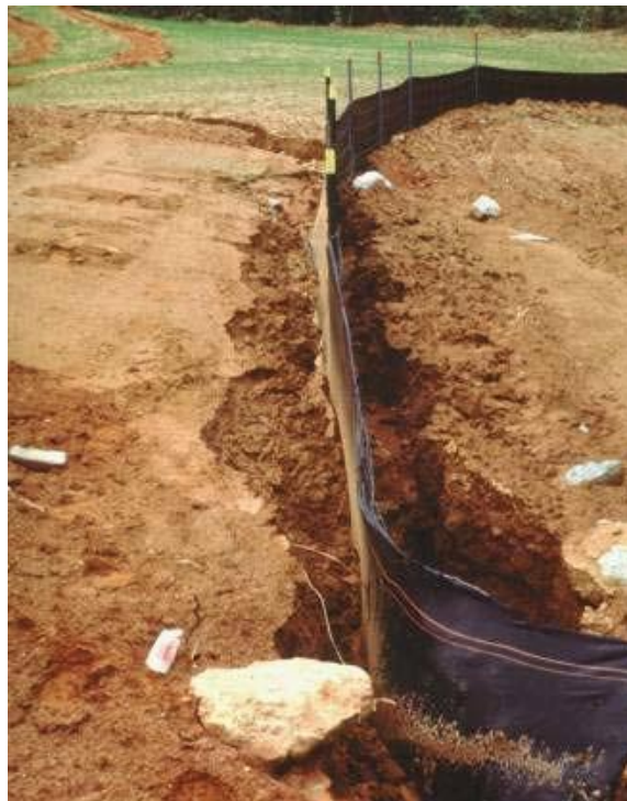
IMPROPER USE OF SILT FENCE AS DIVERSION
