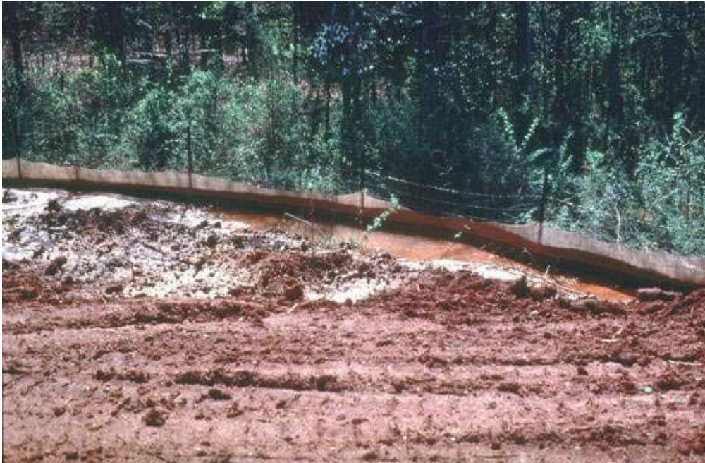
PROPERLY INSTALLED SILT FENCE WITH HEAVY SEDIMENT LOAD. STONE OVERFLOW SHOULD HAVE BEEN INSTALLED.
