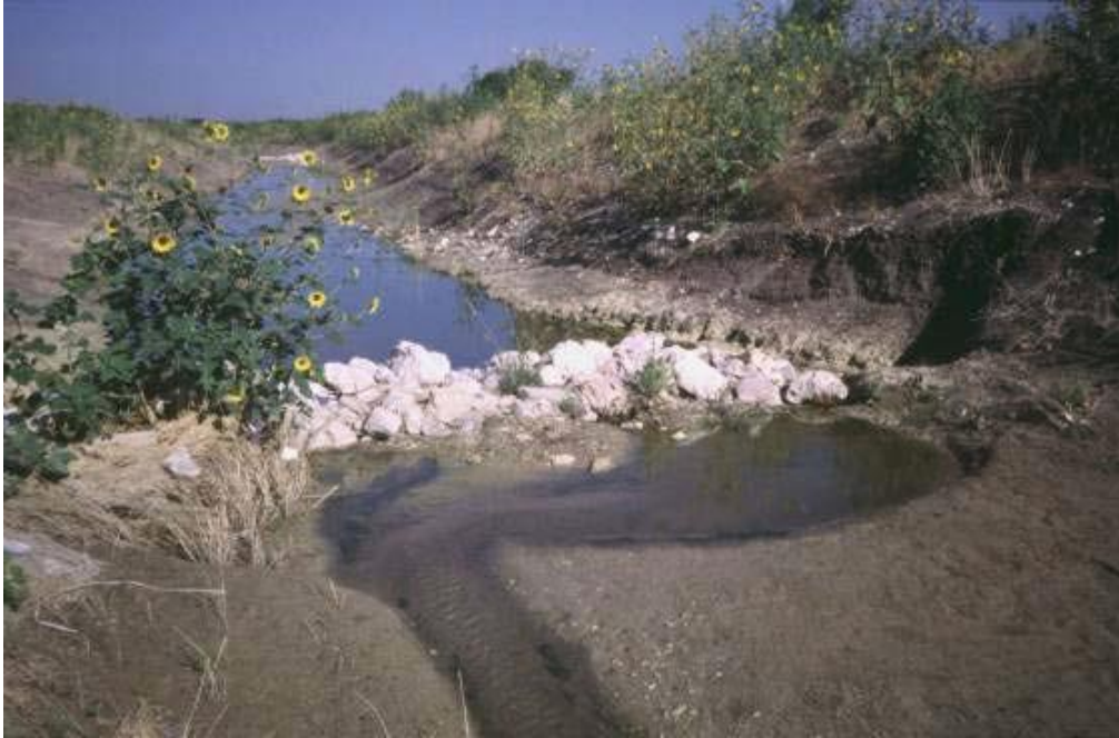
IMPROPER CONSTRUCTION LEADING TO BANK EROSION
