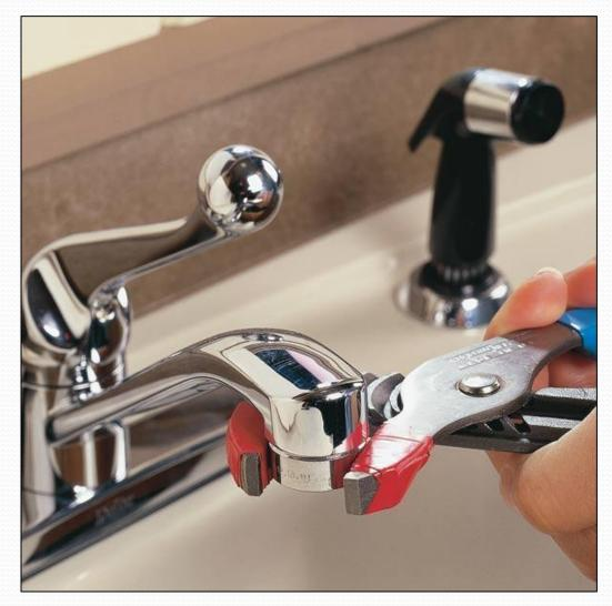
Remove existing aerator if replacing. Use channel locks or crescent wrench to loosen.
