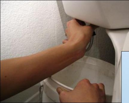
Disconnect the water supply line, unscrew the fill valve locknut. Turn off the water supply, flush the toilet, and sponge the remaining water from the tank.
