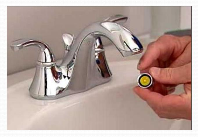
Install new aerator and tighten by hand. Use channel locks or crescent wrench to tighten once quarter turn more.
