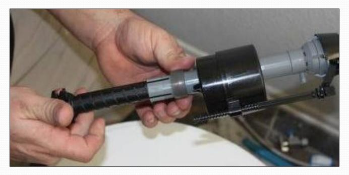
Prepare the new fill valve by adjusting the height of the fill valve as necessary.
