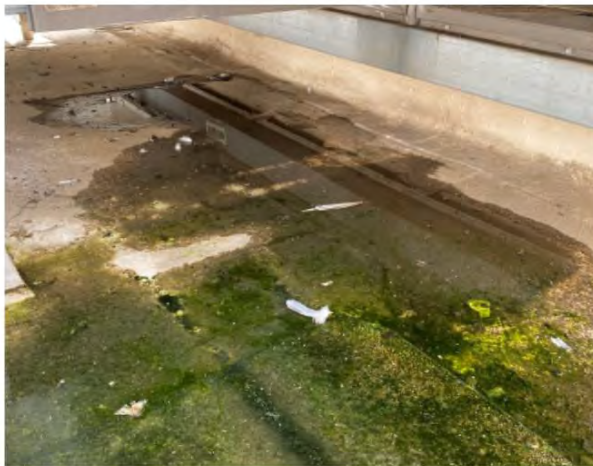
HVAC units on the West roof have improper condensate lines causing water pooling
