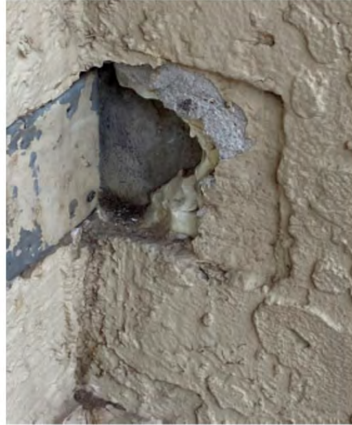
Stucco Damage: Water Entry Points in Recreation Yard
