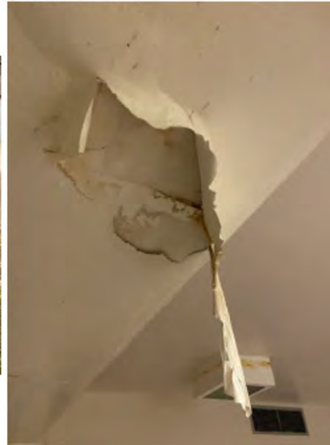
HVAC/Roof issues cause damage to interior ceiling
